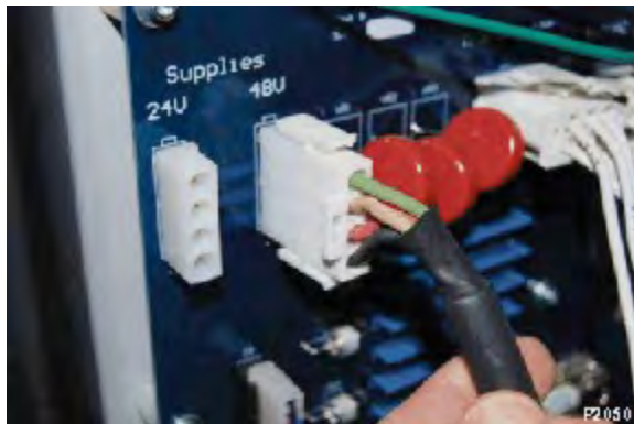
Figure 4-5. Inspection of the cable connections
