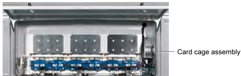
Figure 2-2. Power module assembly
