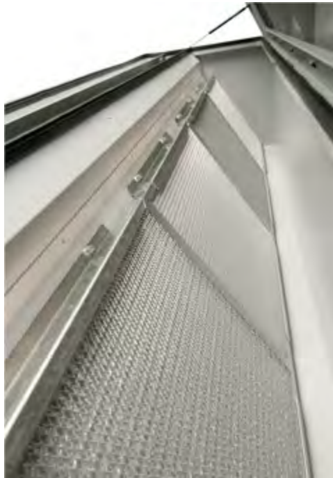
Figure 4-10. Air filter check
